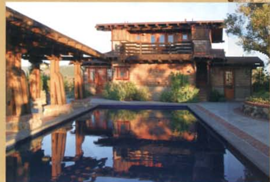
Porches and pergolas take in the sun. A timber-frame sleeping porch off the master bedroom crowns the intersection of the two wings of the house (photo above). Below to its left, the entry gallery is akin to a sidewalk café on the way to the front door. The garage (photo left) is topped by a guest room with a balcony. Photos taken at A and B on site plan.
